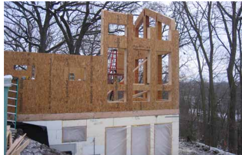
Blunk Residence – SIPA Building Excellence Award Winner Insulspan SIP System
