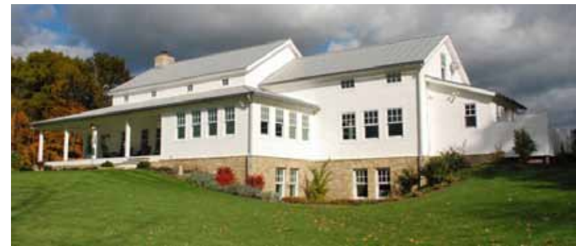
Columbus Home – salvaged 1862 timber frame Insulspan SIP System
