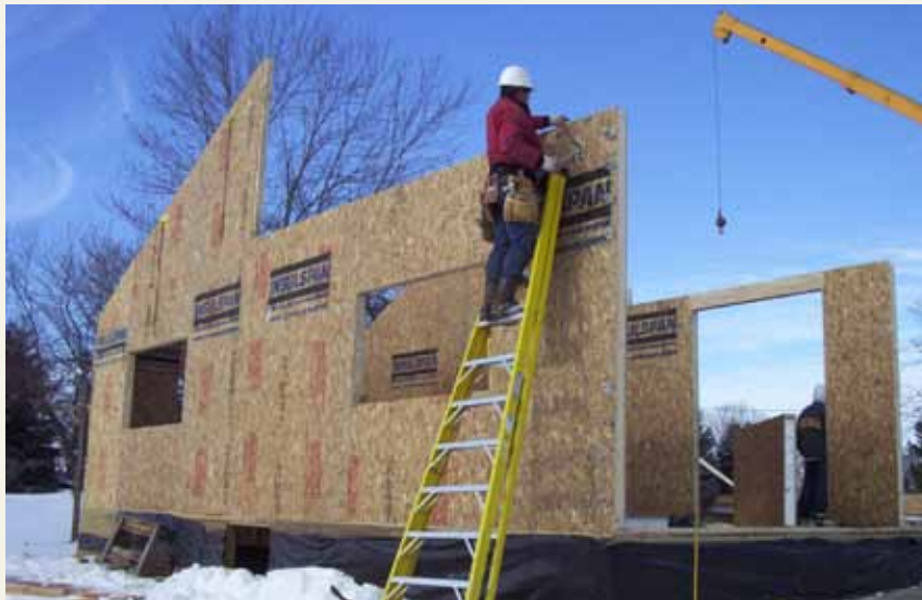
Installing top plates Insulspan SIP System
