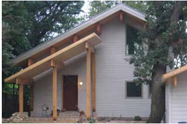
Blunk Residence Batavia, IL 2,680 sq. ft. 0.62 ACH50 HERS Index 42 Insulspan SIP System
