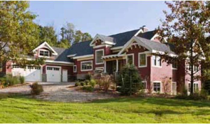
Burnside's Inn (residence) Dexter, MI 4,010 sq. ft. 0.86 ACH50 HERS Index of 37 (includes solar) Insulspan SIP System
