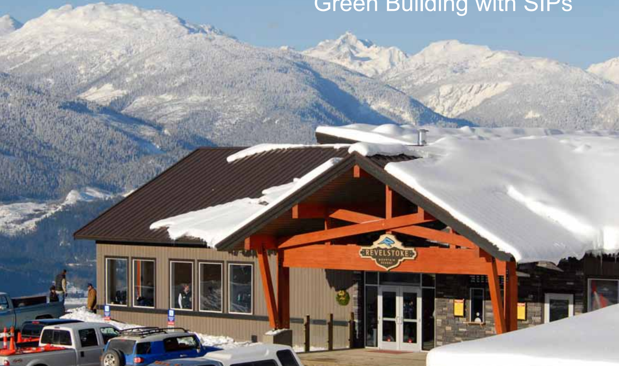
Revelstoke Day Lodge – ski lodge with energy-efficient SIP roof – Insulspan SIP System
