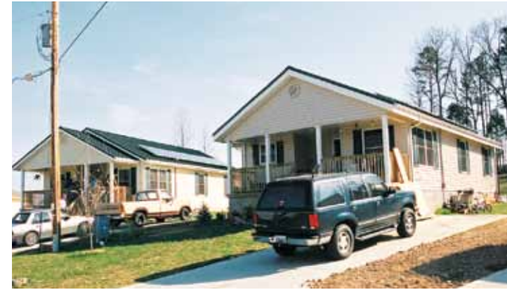
Oakridge National Laboratory Zero-Energy House Lenoir City, TN 2,600 sq. ft. 1.65 ACH50 HERS Index of 45 (includes solar) Insulspan SIP System
