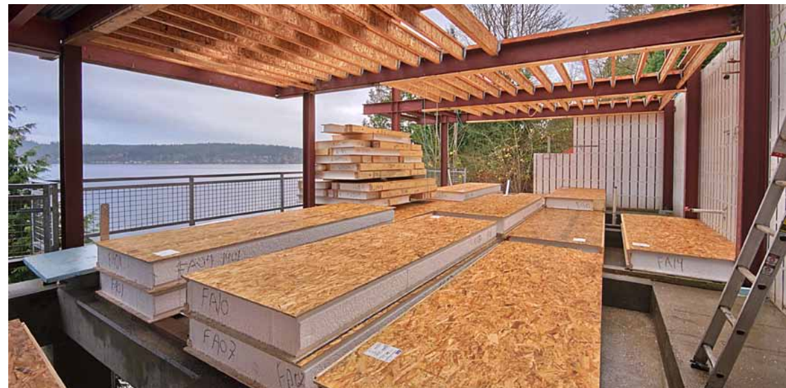
Zero Energy Idea House – a model home for the future Insulspan SIP System
