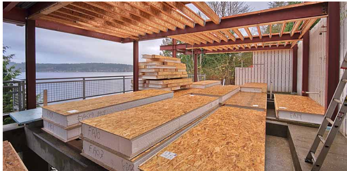
Zero Energy Idea House – a model home for the future Insulspan SIP System
