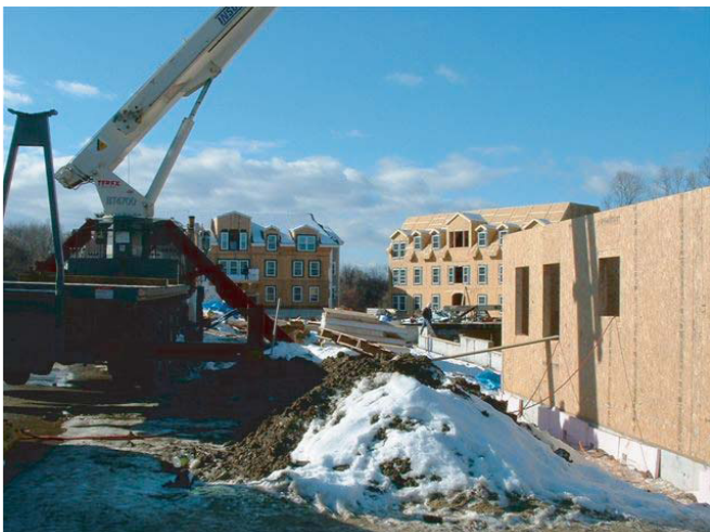
Panels were raised easily with the help of a crane.
