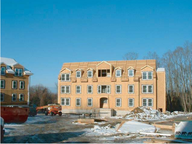
Construction on the buildings was quick and efficient thanks to the prefabrication of the panels and other materials supplied by Panels Pros.
