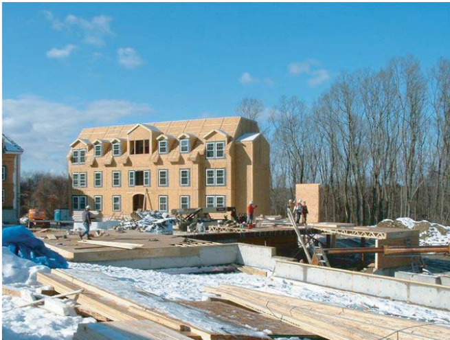
The expansive job site allowed multiple processes of the building to be performed at the same time.
