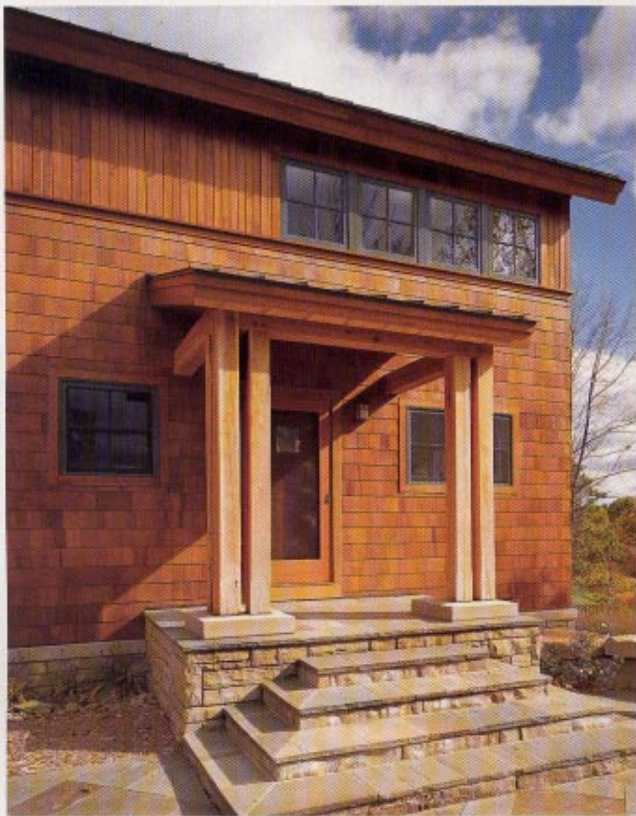
Builder Tim Powell had the vertical cedar tongue-and-groove siding specially milled for the Johnsons' home.
